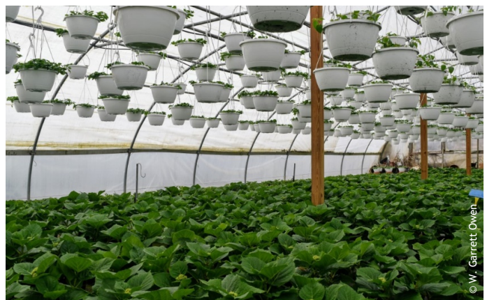
Figure 3. To provide additional support in double poly-covered greenhouses, 2' x 4's can be placed under weight bearing bow and purlin connections, however snow removal may still be required. Photo by W. Garrett Owen.
