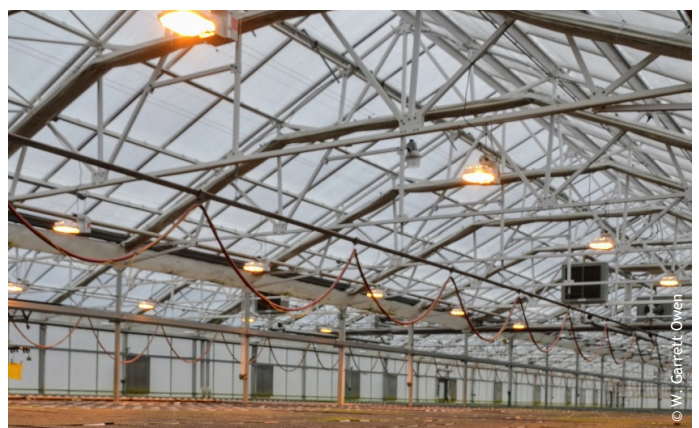
Figure 6. The most common method for melting snow in high-tech glass-glazed greenhouses is to open the energy curtains. Photo by W. Garrett Owen.
