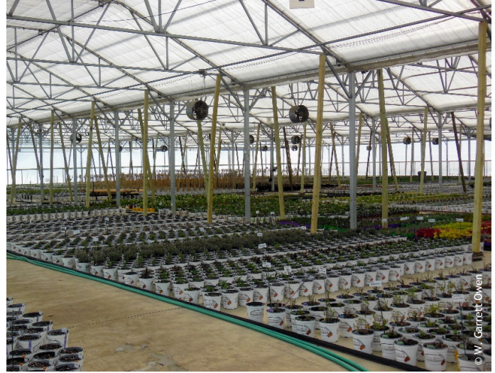
Figure 8. To provide additional support in glass-glazed greenhouses, 2' x 4's can be placed under and near gutter connections, however snow removal may still be required. Photo by W. Garrett Owen.
