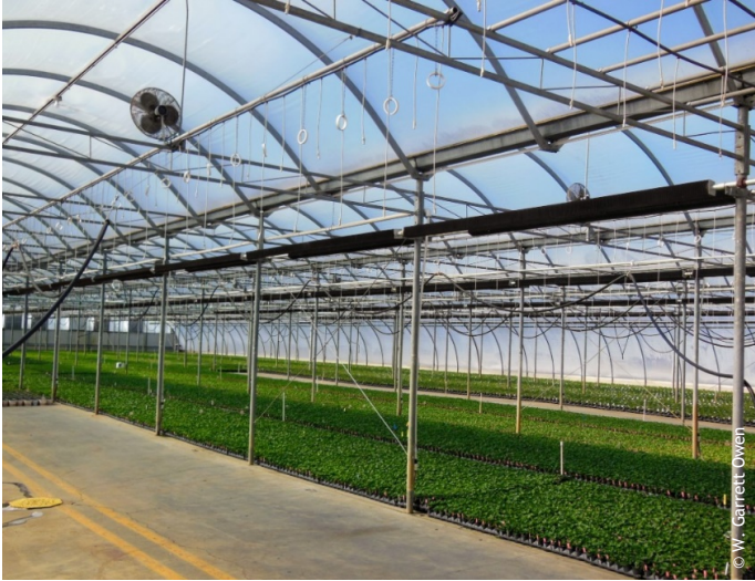
Figure 7. To collapse snow bridging and melt the snow, a heating source such as heating pipes or fins are installed sideways and 18" below the greenhouse gutter. Photo by W. Garrett Owen.
