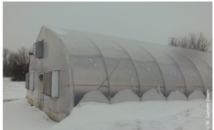
Figure 2. Avoid snow accumulation along the sidewall as it may crush it in. Photo by W. Garrett Owen.
