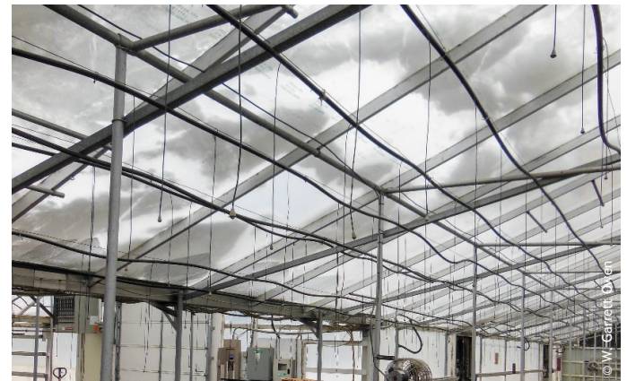
Figure 5. The greatest snow removal challenge is with double poly-covered greenhouses. Photo by W. Garrett Owen.
