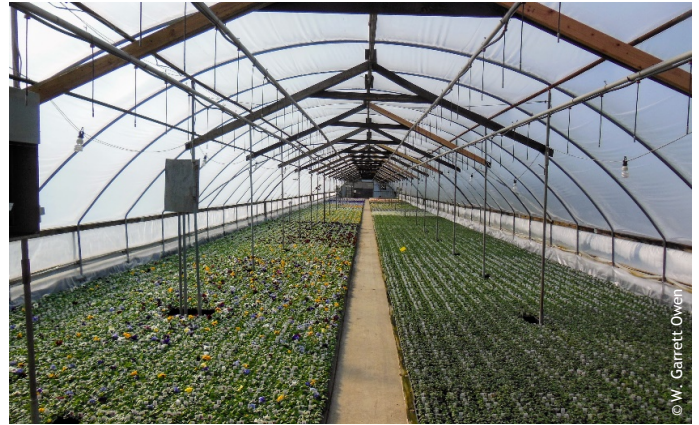
Figure 4. Installation of diagonal braces attached at the peak inside the greenhouse and at vertical supports will provide additional support to the greenhouse structure. Photo by W. Garrett Owen.
