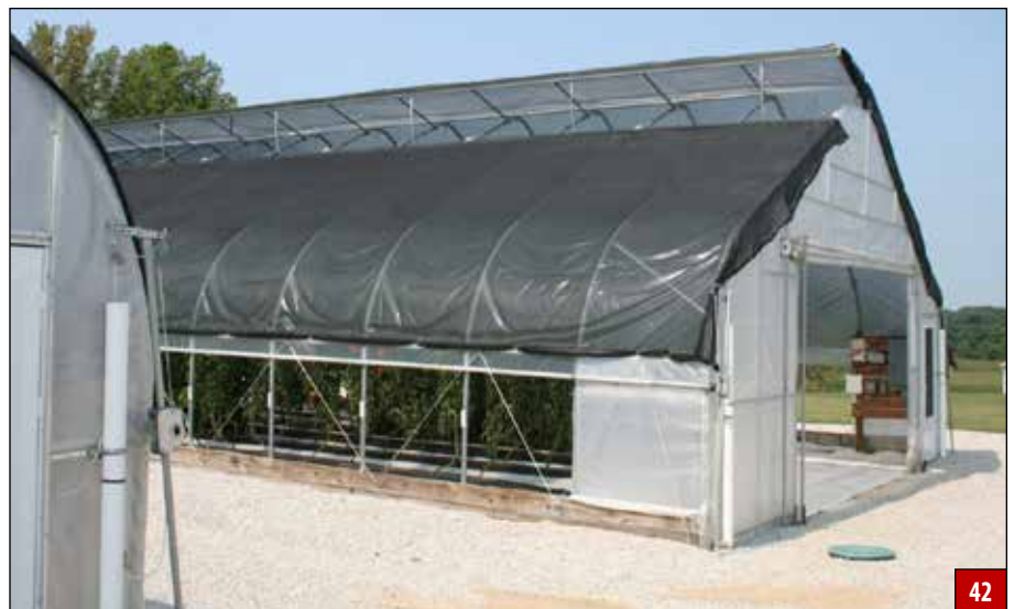
Gravel on the ground surrounding structure exterior.
