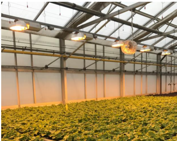
FIGURE 11. Plants grown under natural solar radiation with the addition of supplemental light from a horticultural lighting source.
