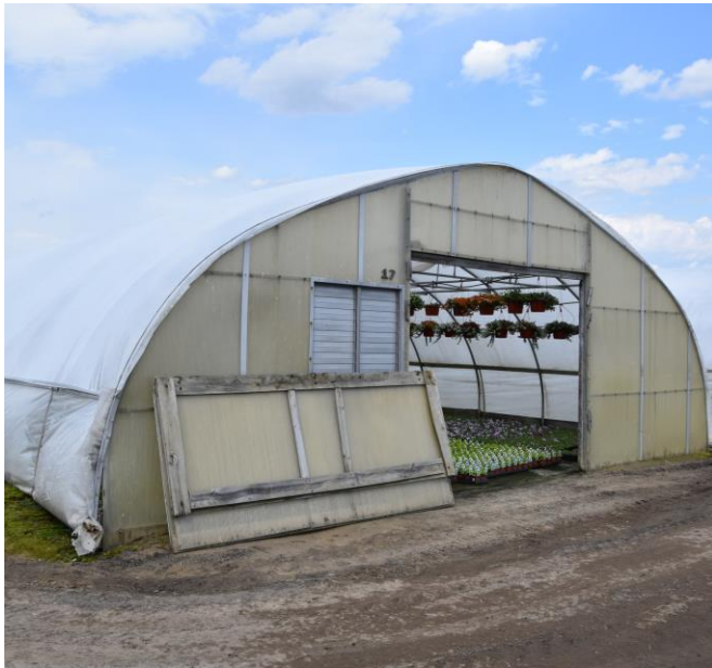
FIGURE 3. High tunnel constructed with a rolling door so machinery can easily access the growing environment.
