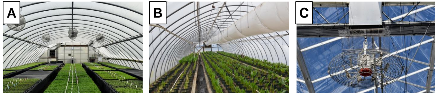
FIGURE 14. In greenhouses, (A) horizontal air flow (HAF), (B) vertical air flow fans, and (C) convection tubes are low-cost technologies to distribute heat throughout the growing environment.
