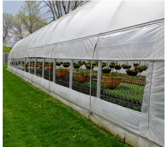
FIGURE 4. Roll up curtains are used to cool or vent the growing environment.
