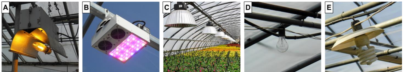
FIGURE 10. Common horticultural lighting technologies include (A) high-pressure sodium (HPS) lamps, (B) light-emitting diodes (LEDs), (C) metal halides (MH) lamps, and (D) incandescent and (E) compact fluorescent bulbs.
