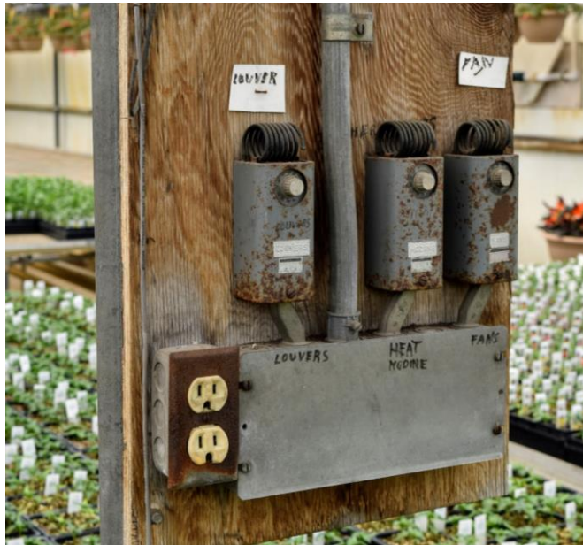
FIGURE 5. In greenhouses, thermostats are often used to manage heating and cooling of the growing environment.
